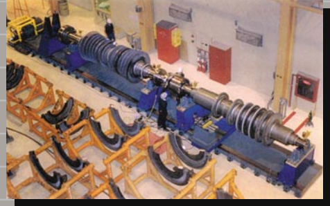
Multiple turbine rotors can be removed and machined while coupled, reducing outage time and improving the consistency of machined surfaces.
