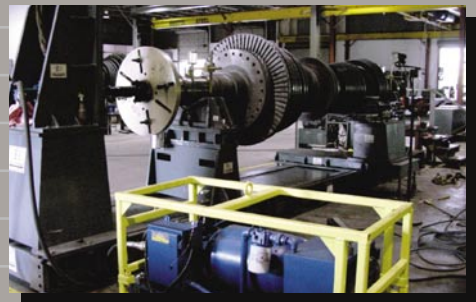
Journal and coupling face machining is conducted using portable lathes with up to 100 tons capacity to remove out-of-roundness and scoring.
